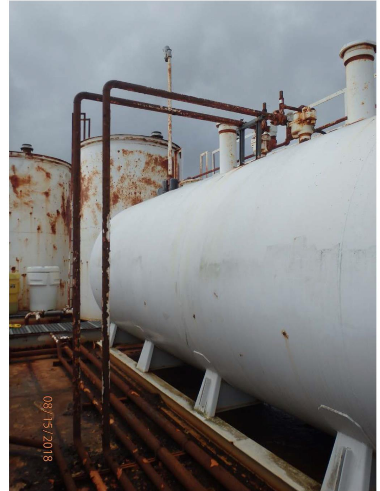
Typical tankfarm piping condition showing complete coating failure and generalized corrosion.
